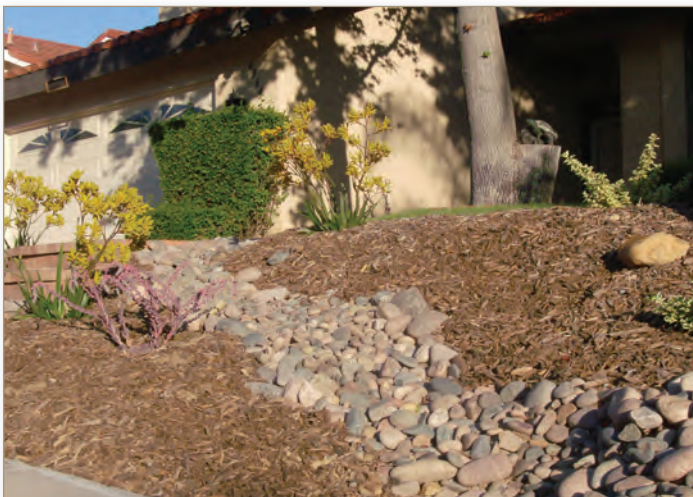
Dry creek beds can be used during wet weather for infiltrating rain water.
