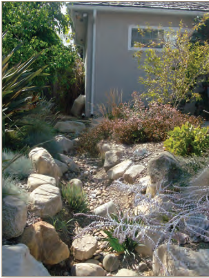
Redirected downspout drain into a landscaped area.
