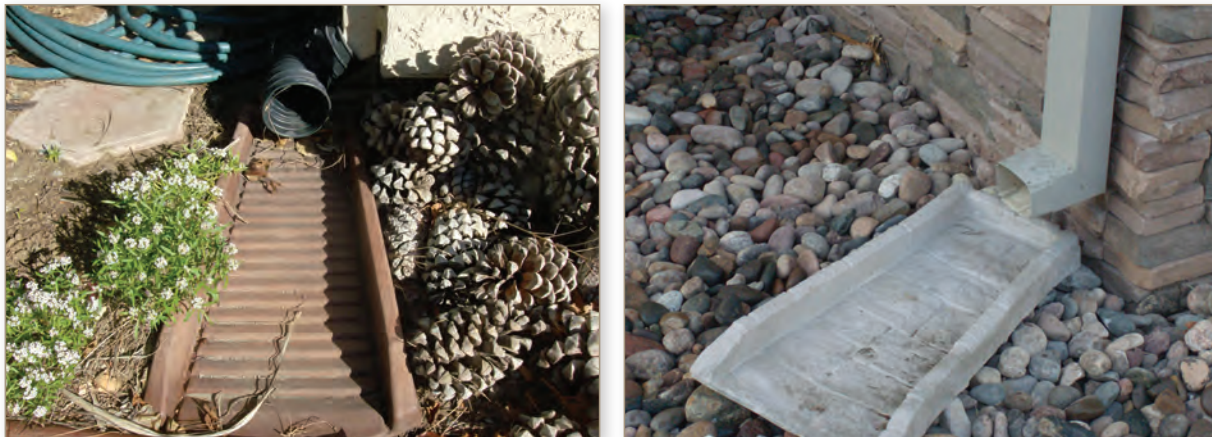
Figure 3-2 Types of Energy Dissipators/Splash Blocks
