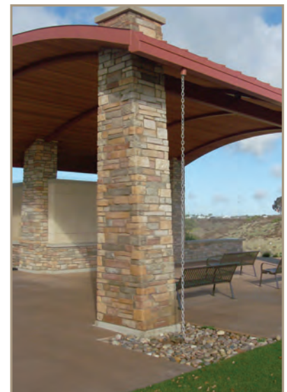
Rain Chain instead of downspout on a San Diego structure
