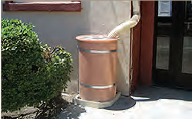
A 55-gallon rain barrel at San Ysidro Library.
