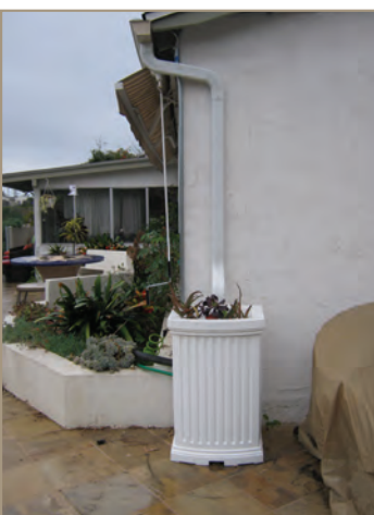
A 50-gallon rain barrel with overflow to a planter box.
